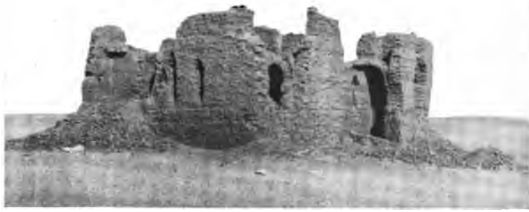
(a) View from southwest.
